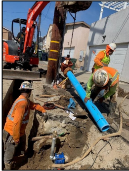
Water Line Installation
