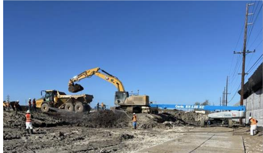
Excavation activities in the northeast area, February 2025
