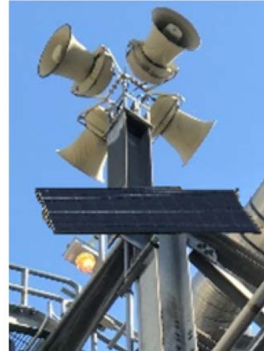
Structure Mounted 1600W High Powered Speaker Stations (4) with • 4 Strobe lights • 4 Solar Panels
