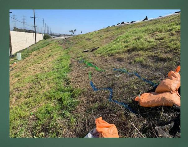
DTSC & ASCON HAVE EVALUATED TENSION CRACKS ON THE NORTHWEST BERM
