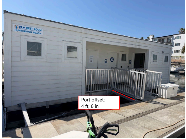
Photograph 8 Port Side of Floating Restroom
