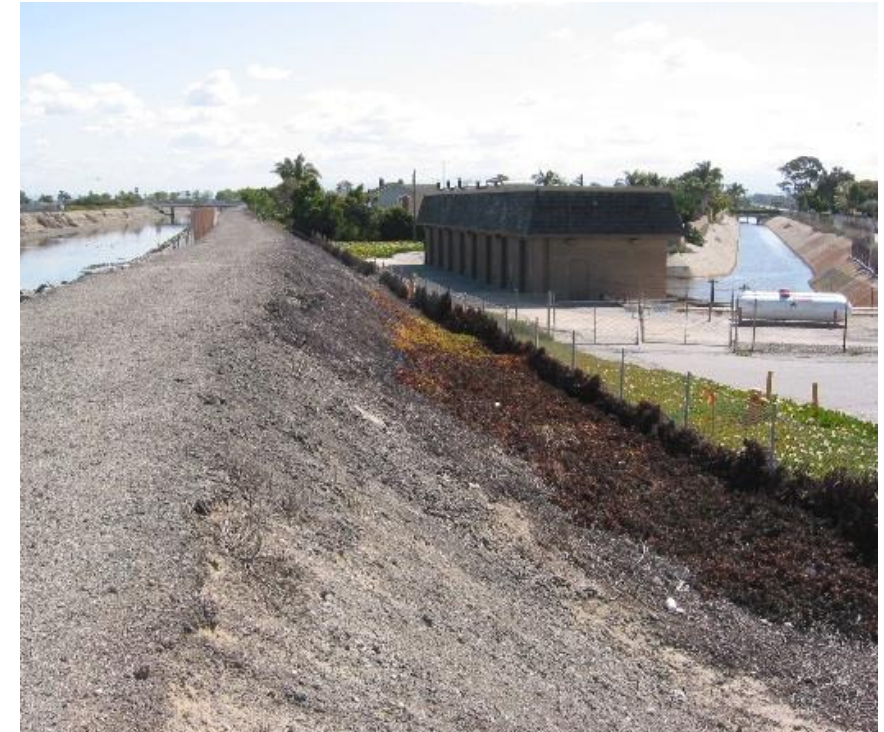
15 Flood Control Stations
