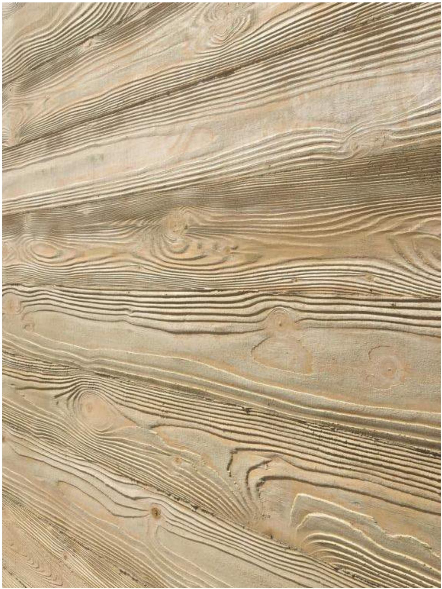
BOARD-FORMED POURED-IN-PLACE CONCRETE
