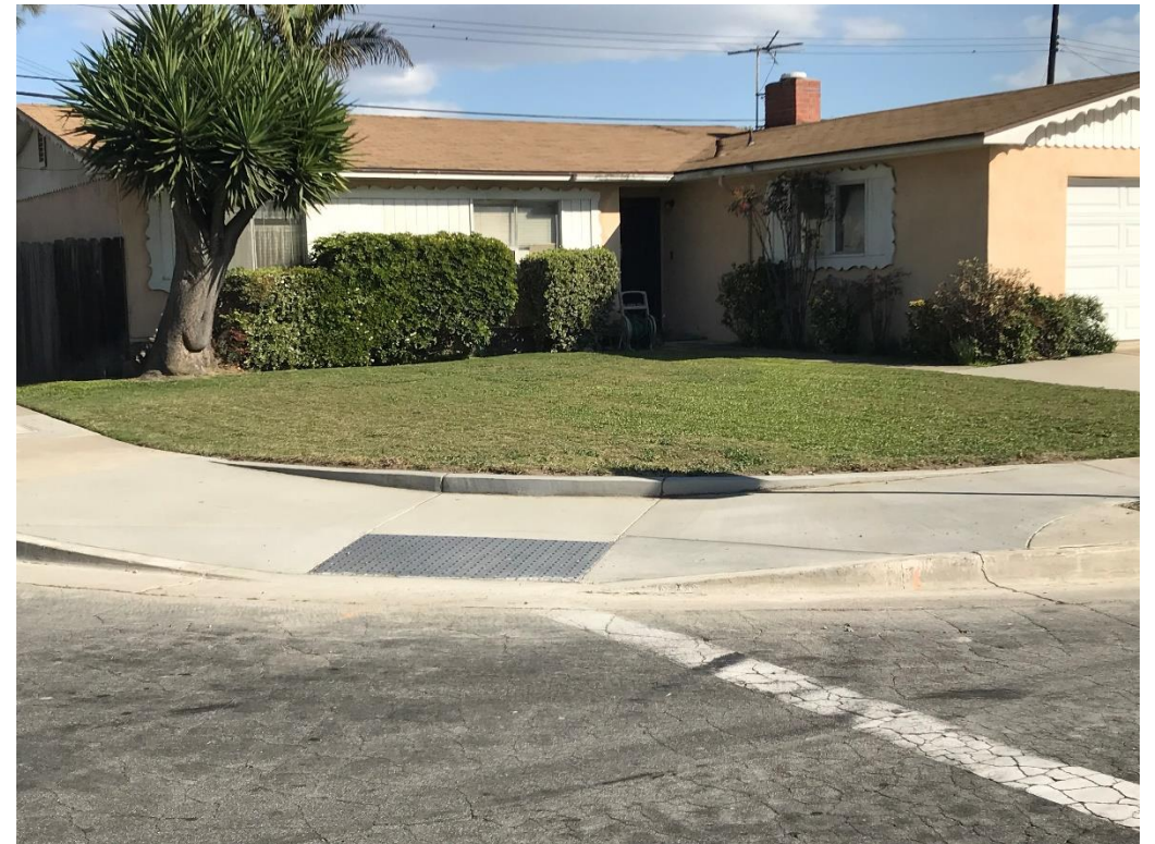
Completed Curb Ramp
