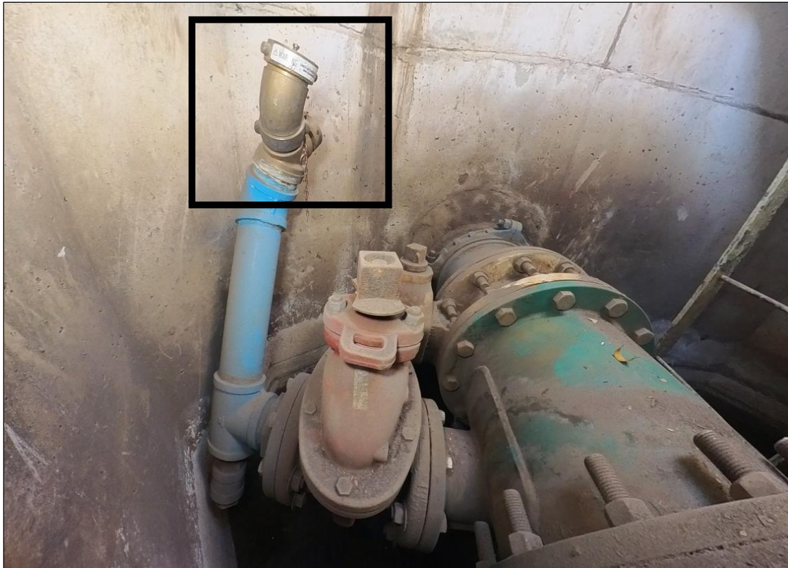
Figure 2: Fire-threaded tap in vault at Westminster Blvd and Springdale St
