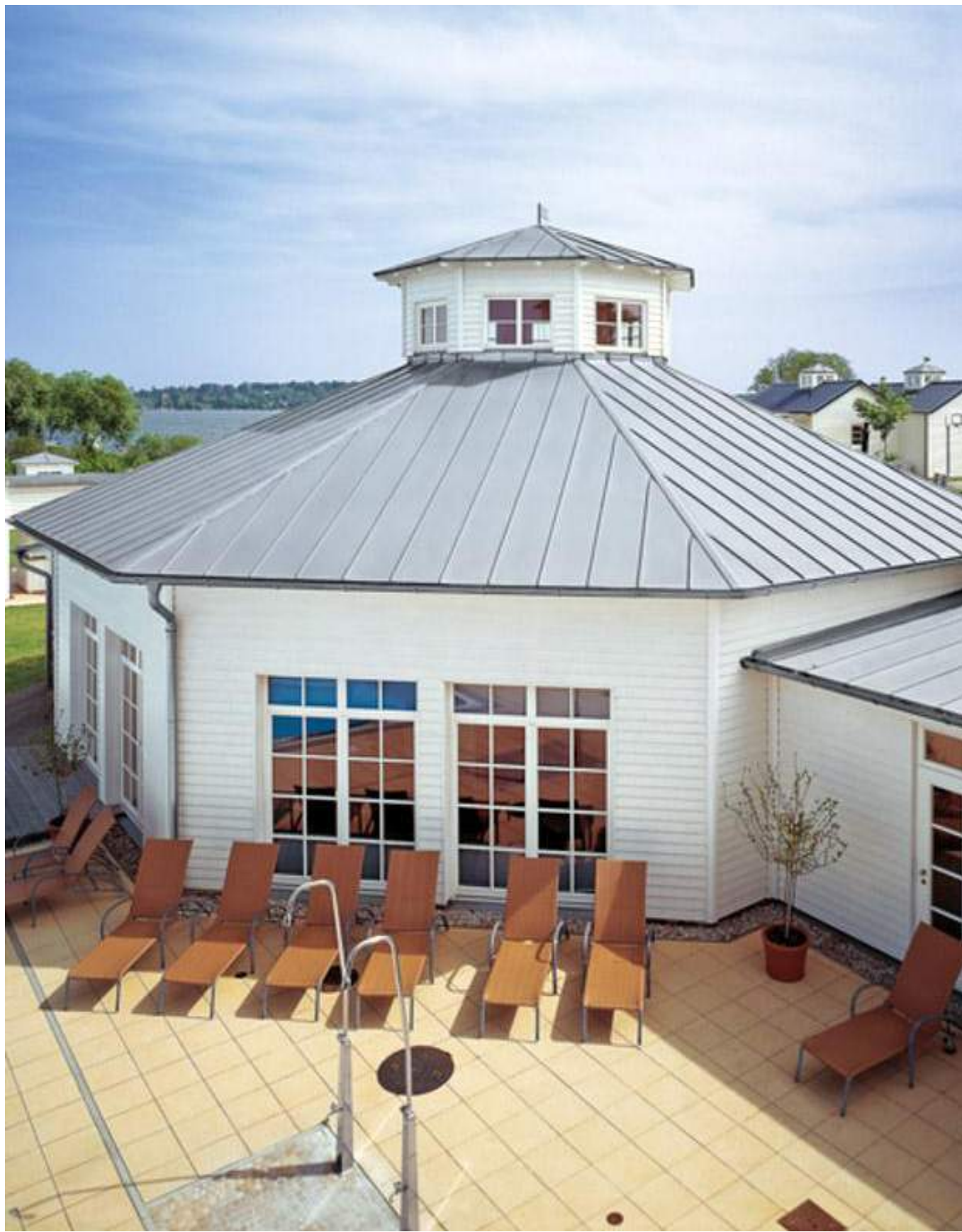
STANDING SEAM METAL ROOFING
