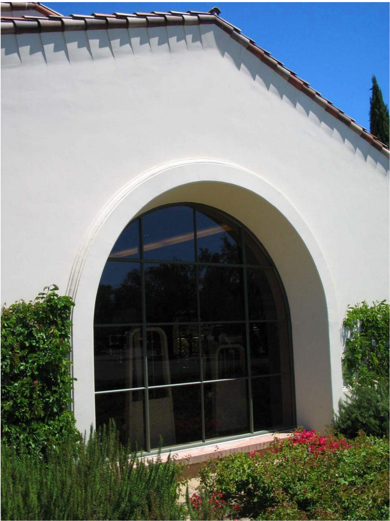
SMOOTH STEEL-TROWLED EXTERIOR PLASTER
