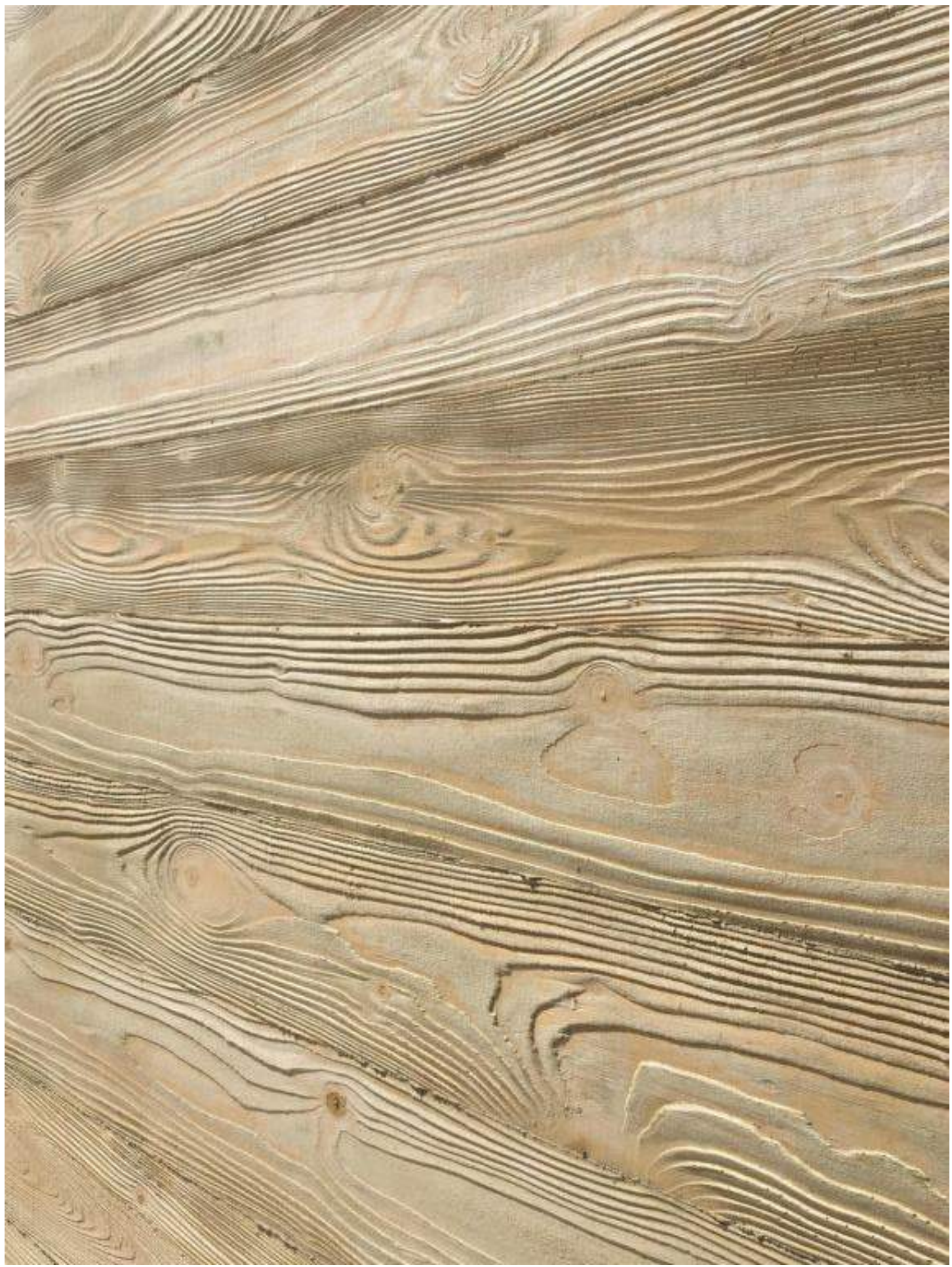
BOARD-FORMED POURED-IN-PLACE CONCRETE
