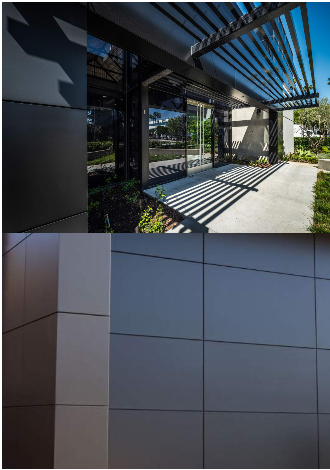
ACM EXTERIOR PANELS
