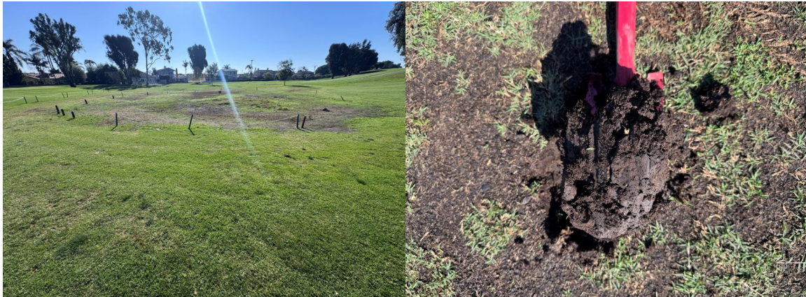
This low area on No. 14 is just 20 yards in front of the green, making this area unplayable. The soil (right) consists of heavy clay which is very slow to drain.
