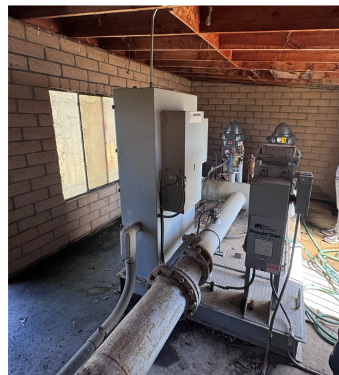
The pump station is in good working condition and is in an acceptable enclosure.
