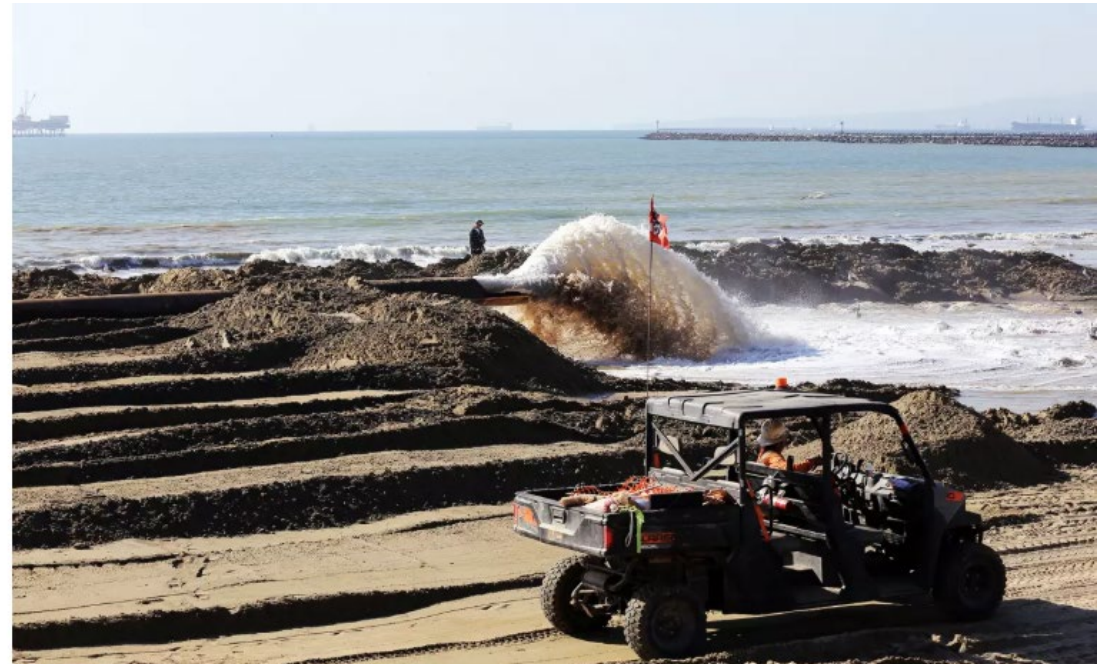
Sand is pumped from a ship two miles offshore in Sunset Beach as part of the sand replenishment project. (James Carbone)
