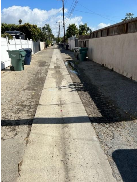
Indianapolis Avenue Alley (2024)
