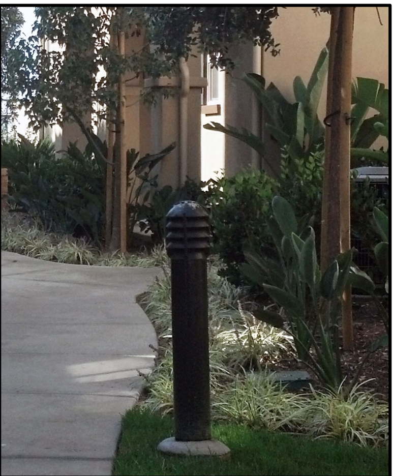
LIGHT BOLLARD Lighting option at walkways where palm/tree uplights, house lighting and street lighting are not sufficient. Light locations are provided for reference only. A photometric study will be provided in the construction document stage to ensure an adequate amount of light fixtures are provided.
