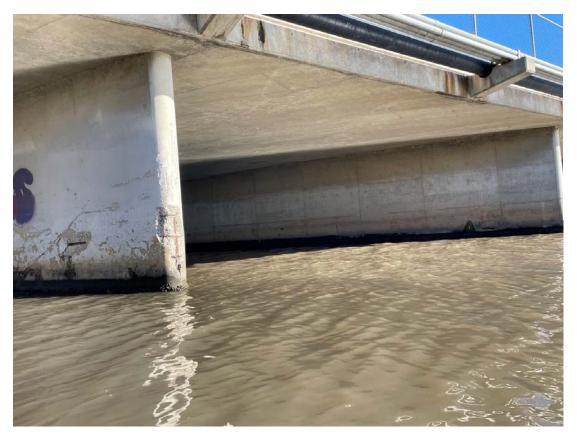
Remove unsound concrete and patch spalls on piers and abutments
