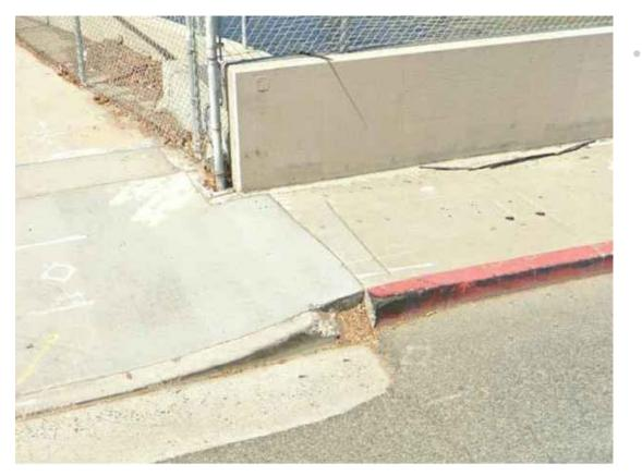
Repair unsound concrete and damaged curb
