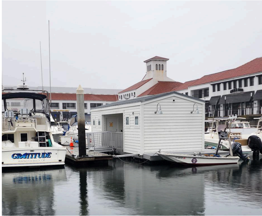
Figure 3 Floating Restroom and Connection to the Dock
