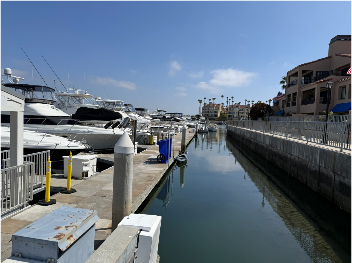
Figure 2 Floating Dock and Concrete Guide Piles at Peter's Landing Marina
