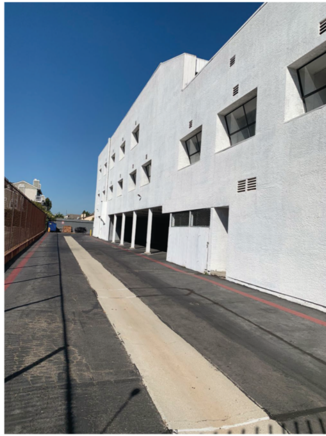
VIEW 4: FULL HEIGHT OF EXISTING PROPERTY (3 FLOORS), FACING WEST
