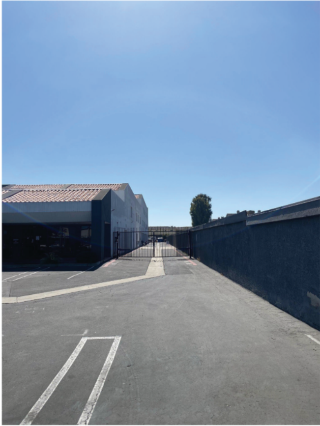
VIEW 16: VIEW OF BACK OF PROPERTY, FACING SOUTH
