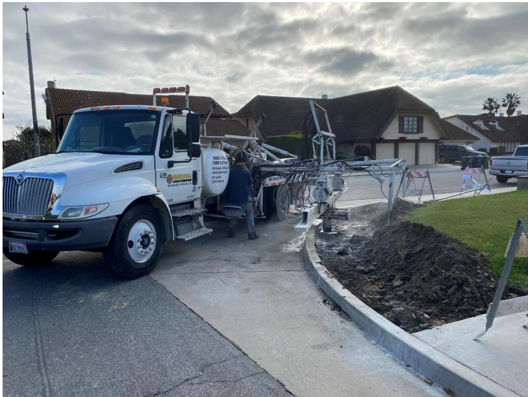
Curb Ramp Construction
