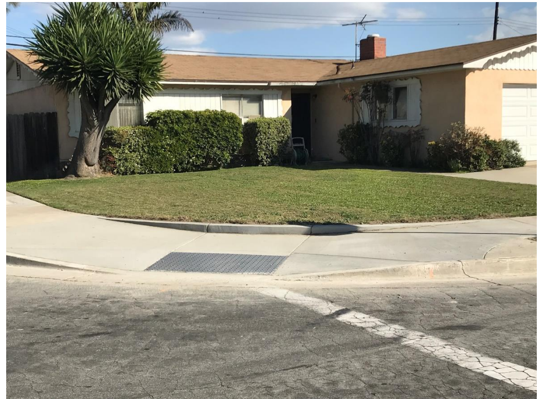
Completed Curb Ramp
