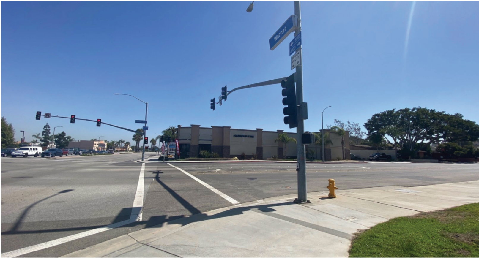
VIEW 8: VIEW OF PROPERTY ACROSS STREET, FACING EAST
