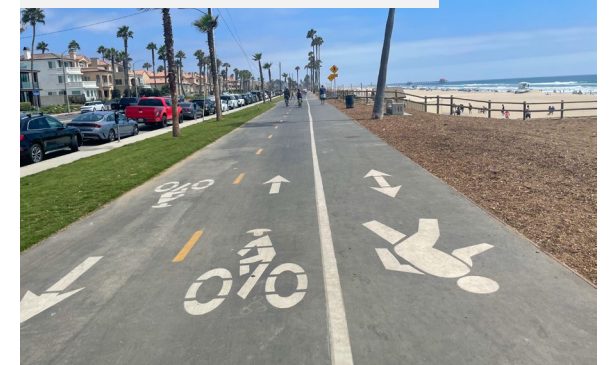
New Path Separation
