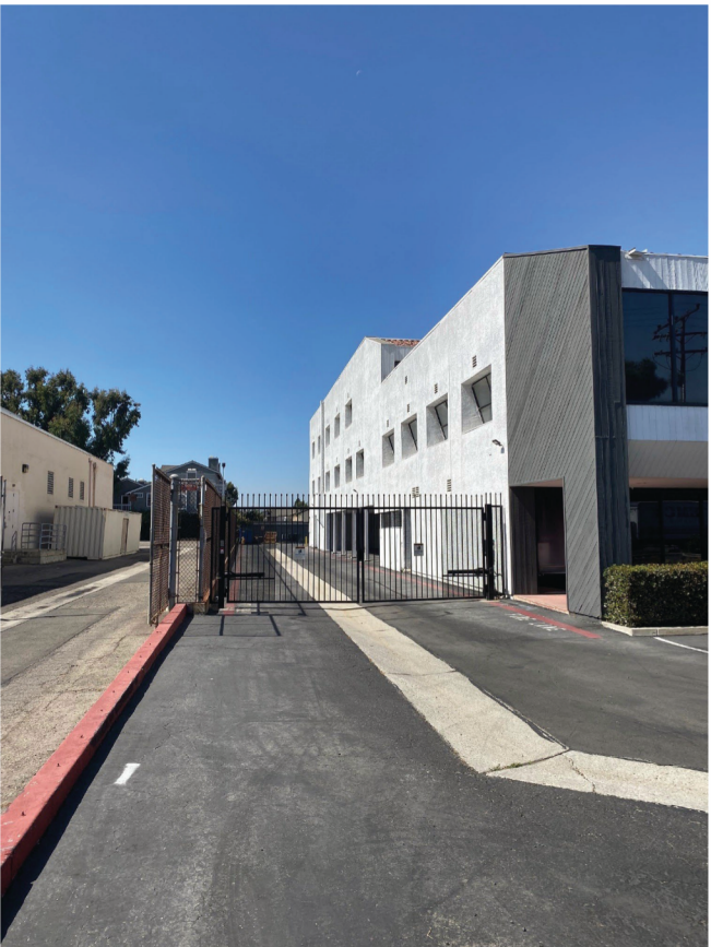
VIEW 3: VIEW OF BACK OF PROPERTY, LOOKING WEST
