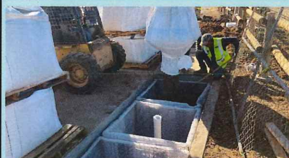
Filling up bio filtration unit with gravel
