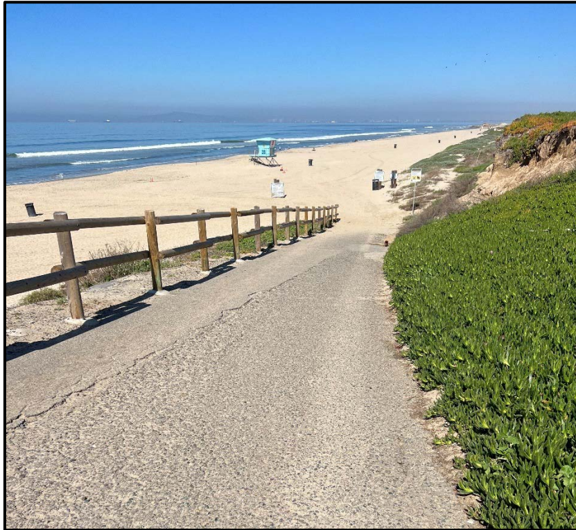
Figure 2.2-3. Access Ramp from Bluff Top Park to Dog Beach
