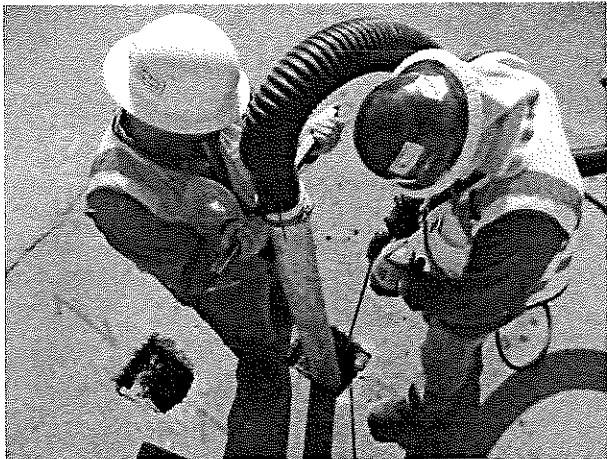
C Below technicians performing potholing
