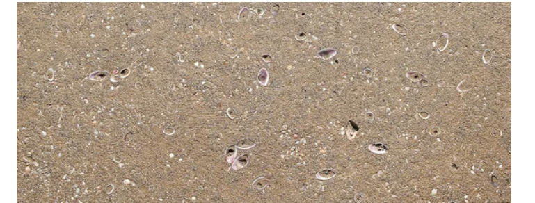
Cast-in-place concrete wall cap in sand color with seashells
