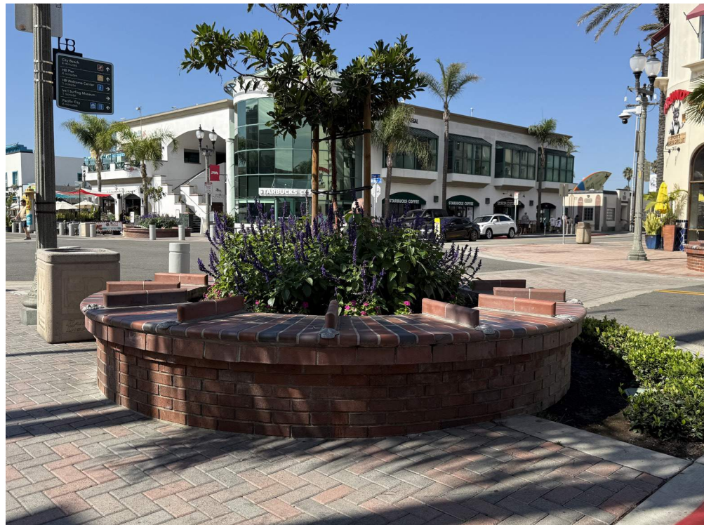
BRICK SEATWALL WITH IN GROUND PLANTER QUANTITY: 10
