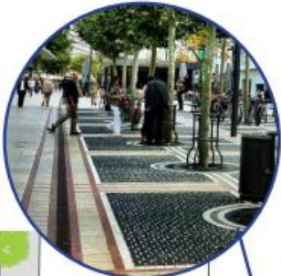
ZERO CURB PLAZA WITH DRAINAGE GRATE
