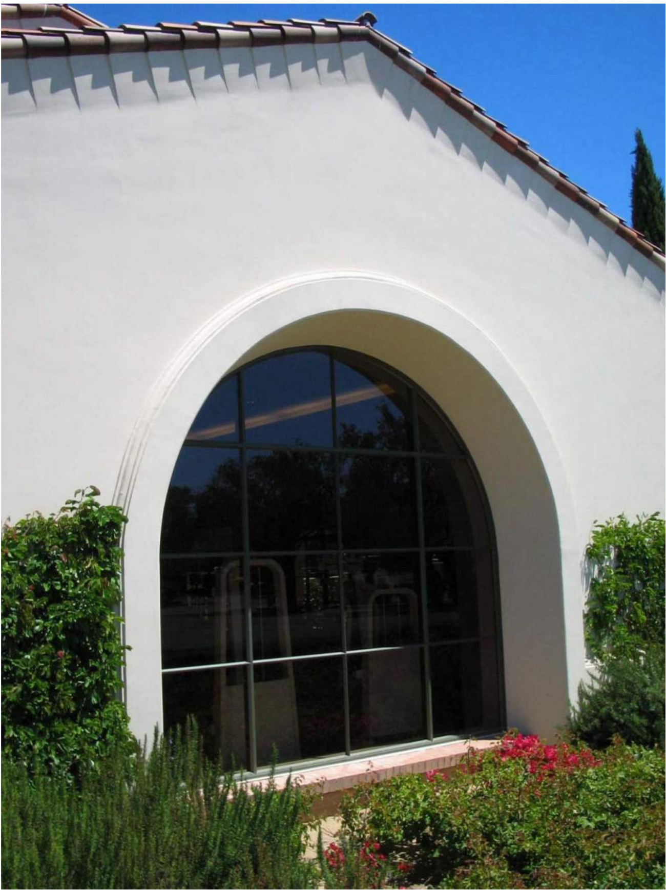
SMOOTH STEEL-TROWLED EXTERIOR PLASTER
