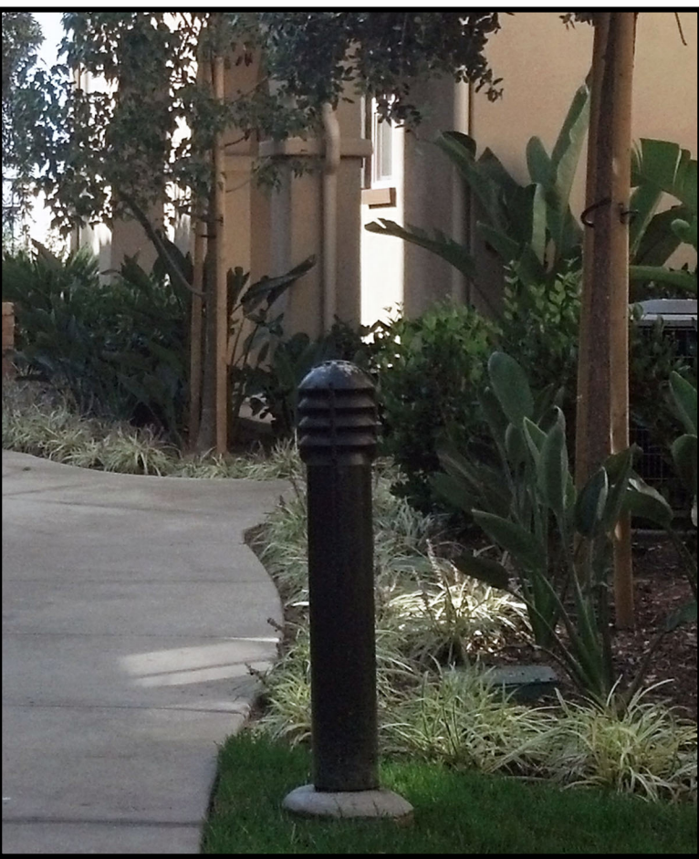
LIGHT BOLLARD Lighting option at walkways where palm/tree uplights, house lighting and street lighting are not sufficient. A photometric study will be provided in the construction document stage to ensure an adequate amount of light fixtures are provided.
