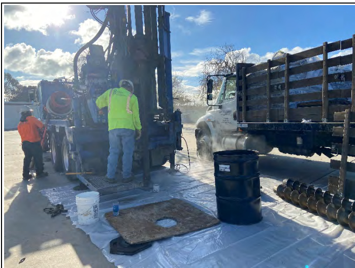
Drilling through concrete slab at HSA-7A (looking southeast)
