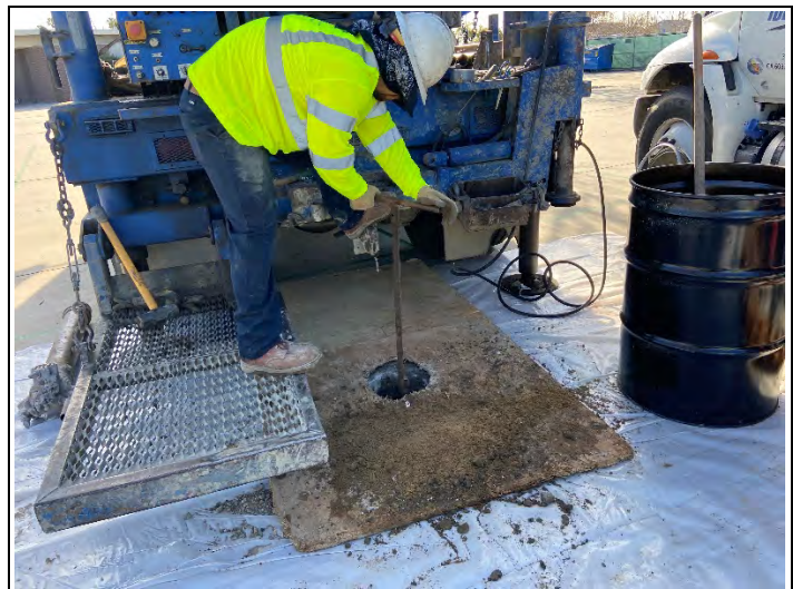
Hand augering at HSA-7A (looking east)
