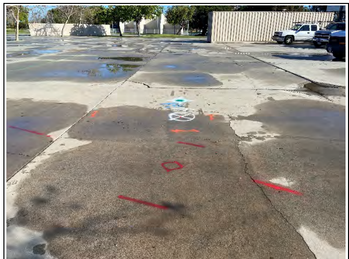
Marked utilities at HSA-4A and the new HSA-4A location (looking north)
