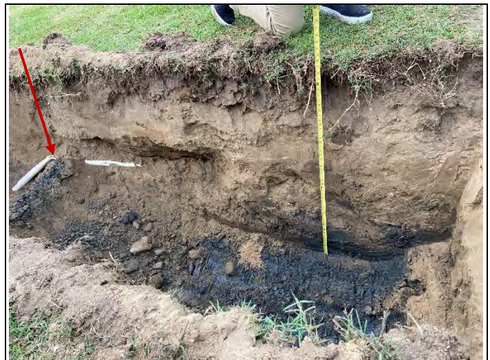
Waste encountered at TP-1. Also indicated is the exposed underground irrigation pipeline (looking southeast).
