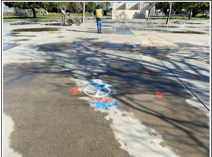
Marked anomalies at HSA-6A and the new HSA-6A location (looking north)
