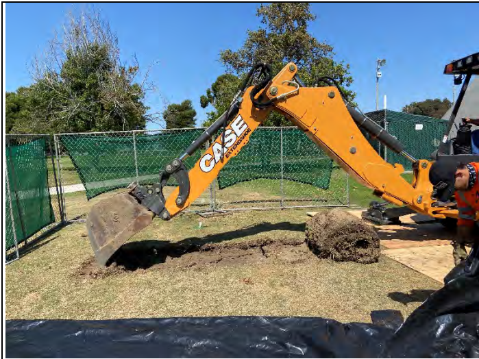
Start of excavation at TP-2 location (looking north).
