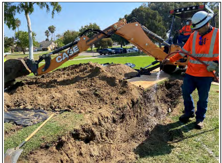
Backfilling at TP-1(looking northeast)
