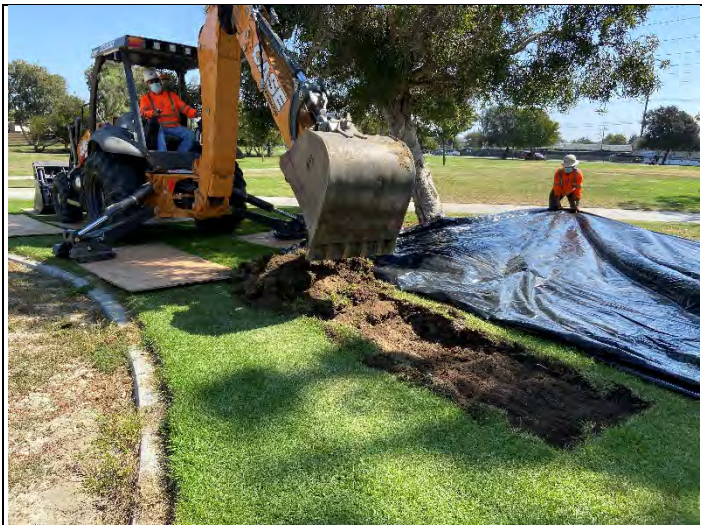
Start of excavation at TP-5 (looking southeast).
