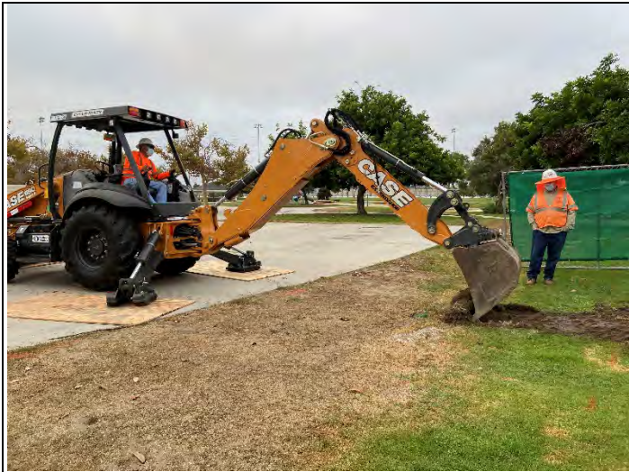
Resumption of excavation at TP-3 location (looking south).
