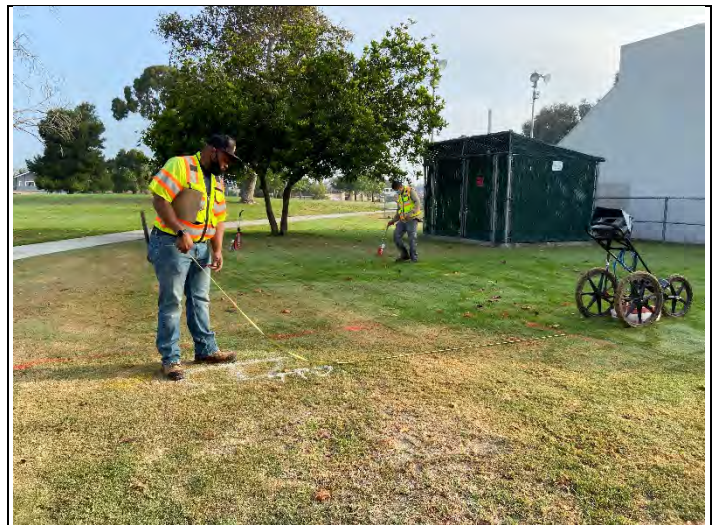
GEOVision crew performing utility clearance survey at location TP-2 (looking north)
