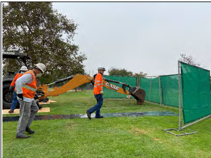
Start of excavation at TP-1 location (looking south).
