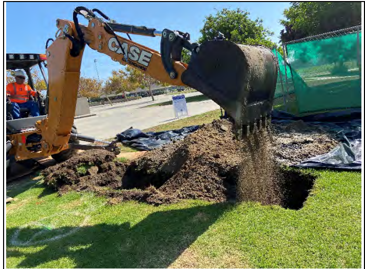
Backfilling at TP-3 (looking southeast).
