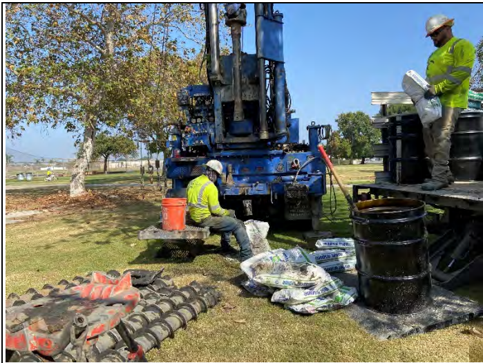
Backfilling the borehole at HSA-5 (looking northeast).
