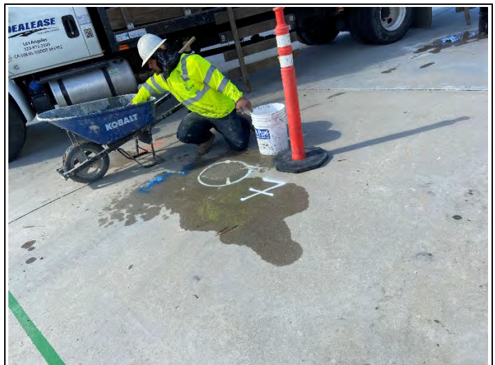
Surface patching with rapid set concrete at HSA-7A (looking southwest)
