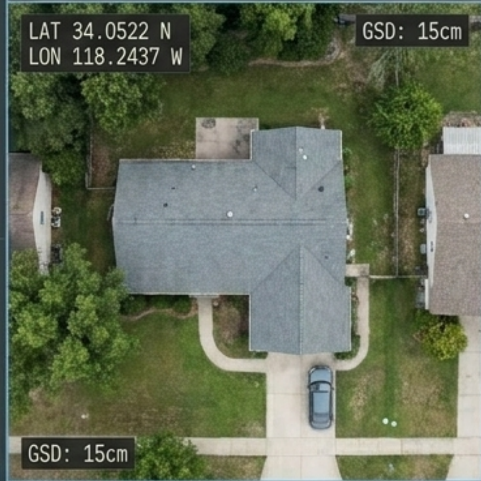
Structural geometry & visible defects.
