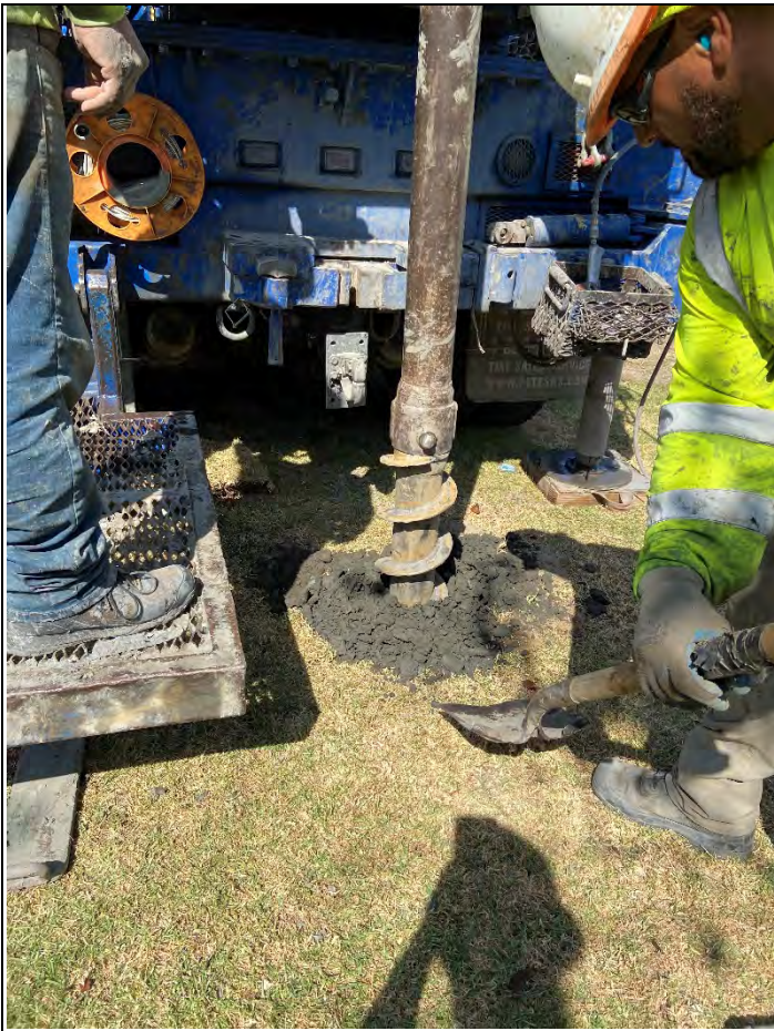
Waste observed in the soil cuttings at HSA-3 (looking northeast).
