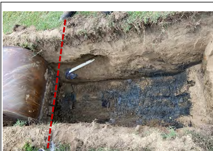
Lateral limit of waste at TP-1 (looking south)
