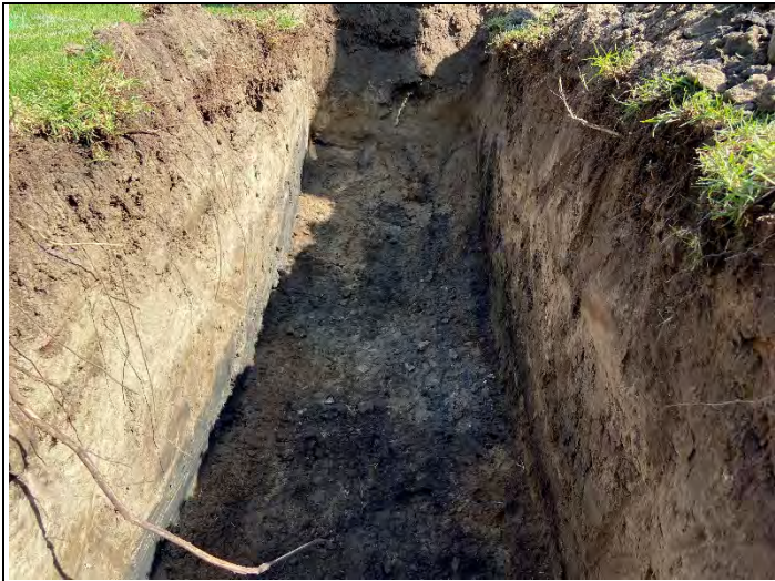
Waste encountered at TP-3 (looking east).
