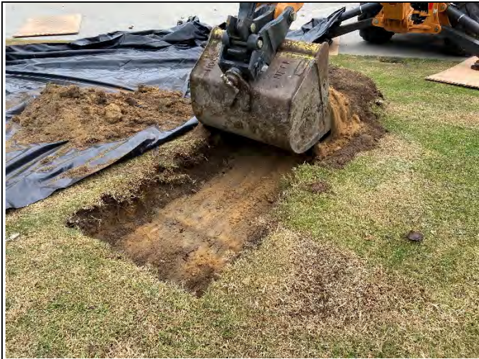
Start of excavation at TP-4 location (looking northeast).
