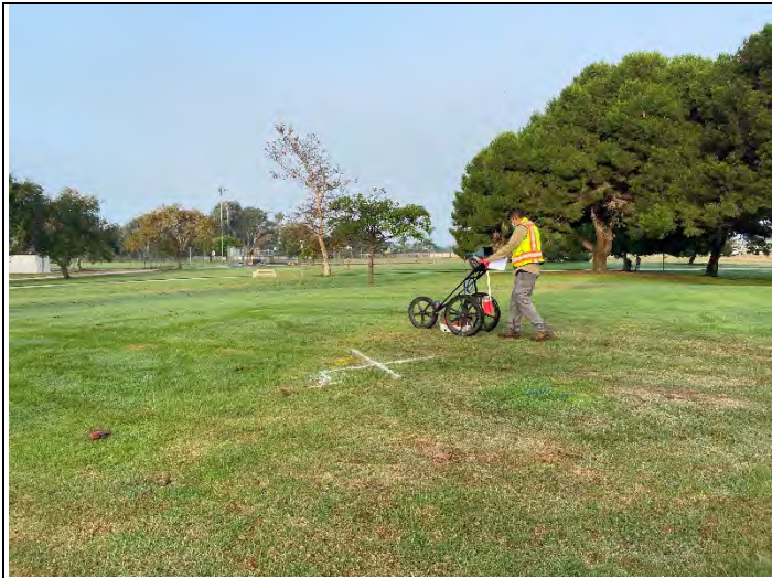
GEOVision crew performing utility clearance survey at location TP-1 (looking west)
