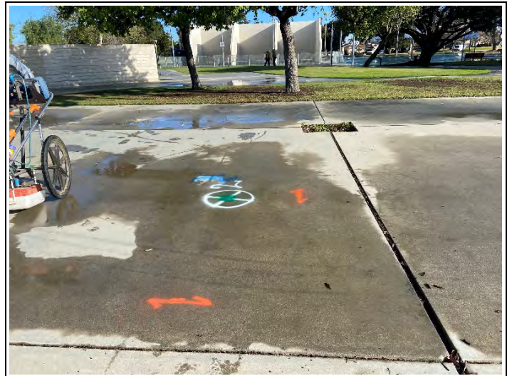
Location HSA-2A cleared of utilities (looking north)
