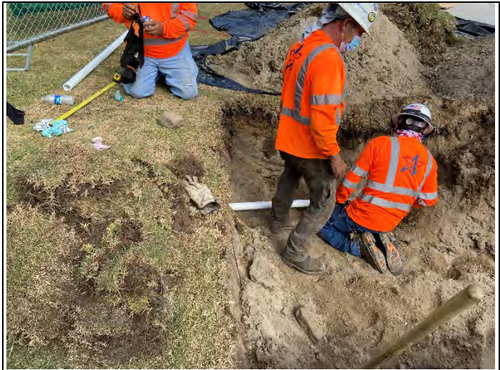
AIS repairing the damaged irrigation pipe at TP-4 (looking northwest).
