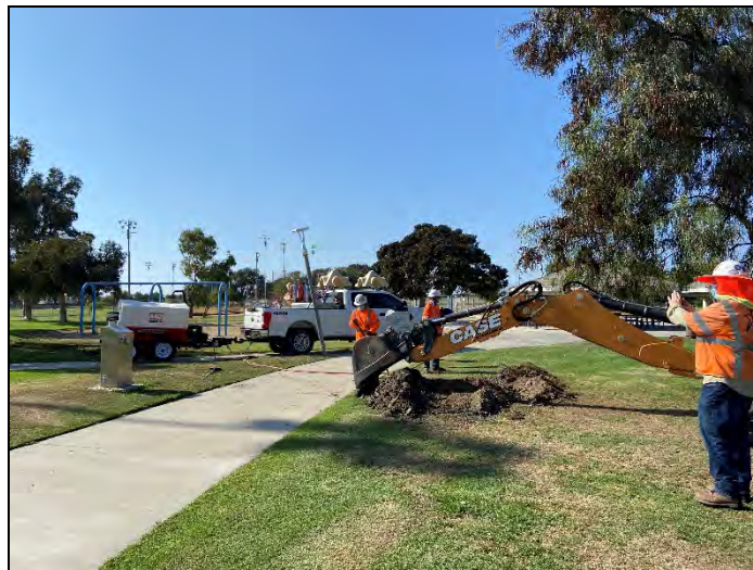
Backfilling the pothole at TP-5 (looking northwest).
