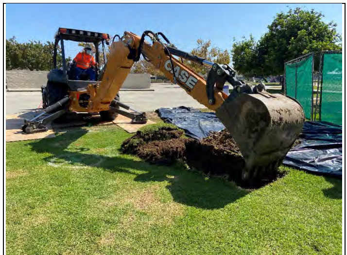
Start of excavation at TP-3 location (looking southeast).
