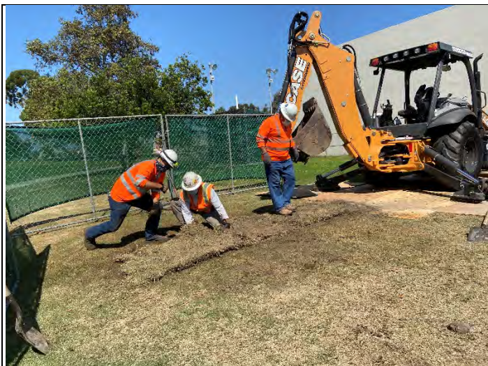
Backfilling at TP-2; placing the vegetation back (looking northeast).
