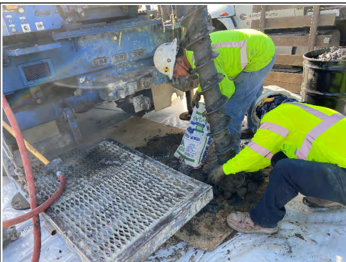
Backfilling the borehole at HSA-7A with hydrated bentonite chips (looking southeast)
