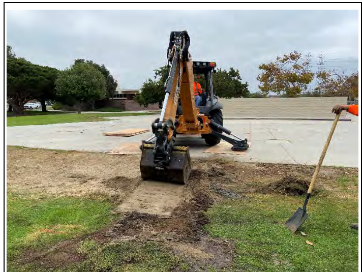
Backfilling at TP-3 (looking east)
