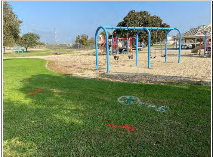
Location TP-5 cleared of utilities (looking northwest). The anomalies located are likely roots.
