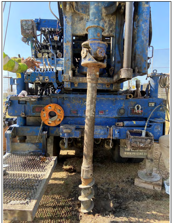
Tilting of auger at HSA-4 (looking west).
