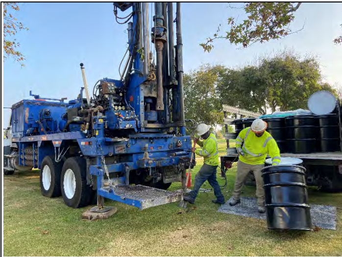
Removal of top soil and vegetation at HSA-5 (looking northeast).
