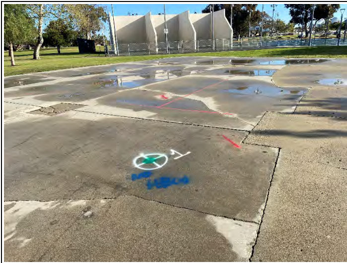
Location HSA-1A cleared of utilities (looking north)
