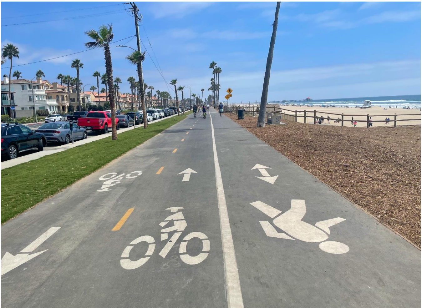
Exhibit 2: Segment 2 - Upper Bluff Path Bicycle and Pedestrian Separation (August 2022); credit Toole Design Group
