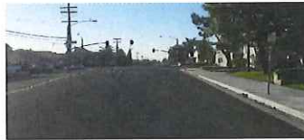
Arterial Rehab – After
