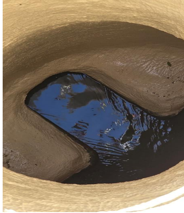
Manhole Rehabilitation
