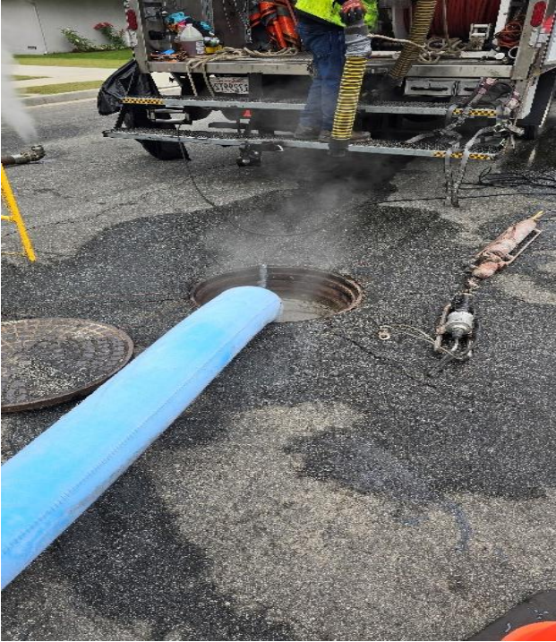
Sewer Lining - Trenchless Technology
