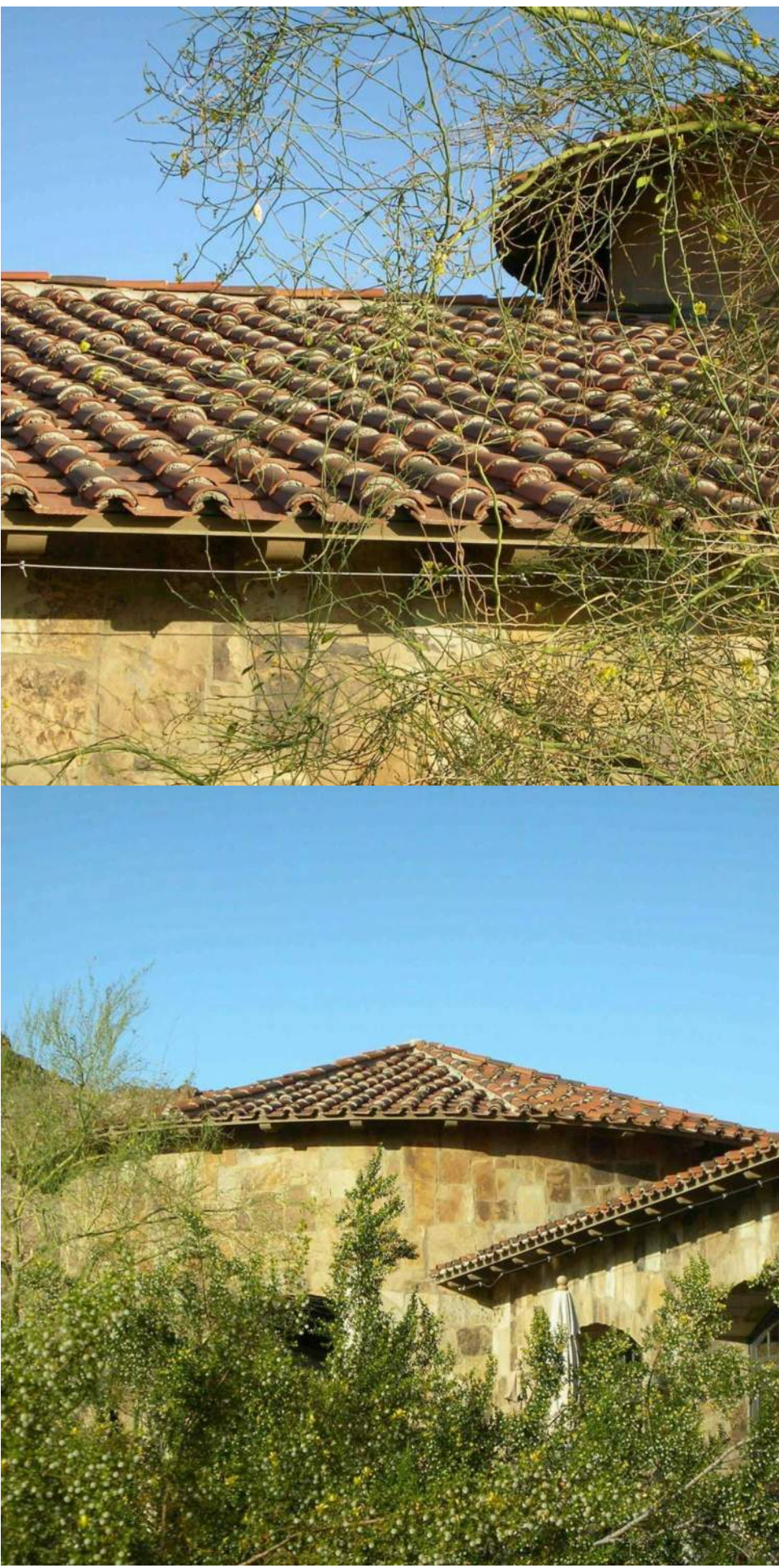
CLAY TILE ROOFING
